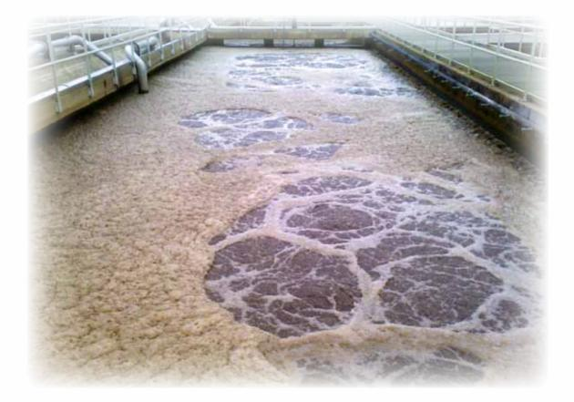
**E**ffluent foaming or excessive foaming in a treatment process is not only a detriment to the discharge quality but also to treatment operations. Often, the application of a defoamer/antifoam is all that is required to eliminate foaming issues.
